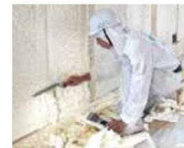
fig.18 削り作業
